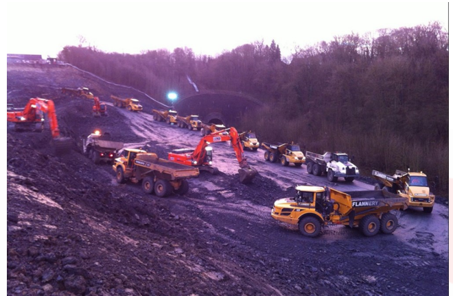
Murphys fleet shifting the material from the cutting to the stockpile
