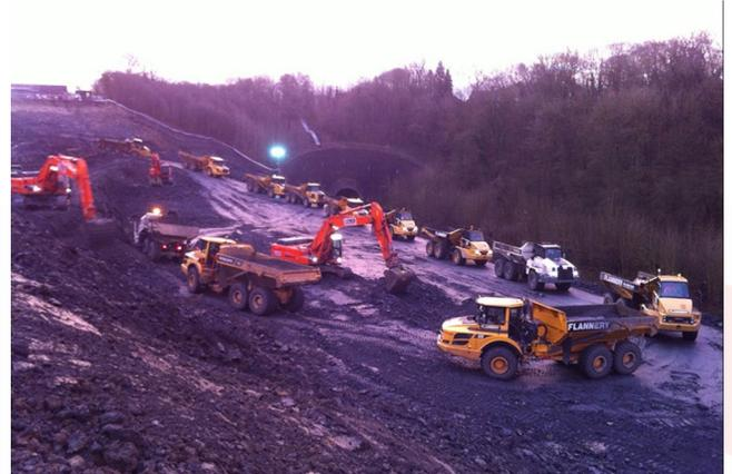
*Murphys fleet shifting the material from the cutting to the stockpile*
